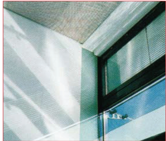
Light redirection system ( Okasolar ). 1
